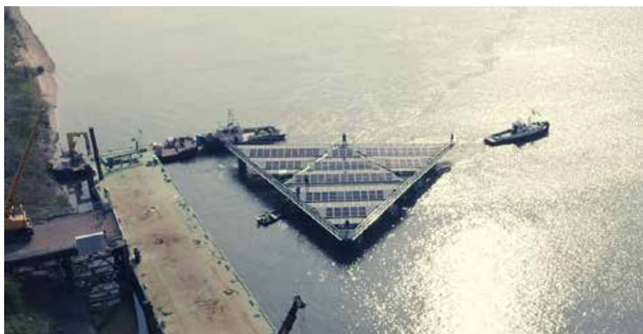
The SolarDuck project Demonstrator floats at IJzendoorn in the Netherlands and delivers energy to the grid.
