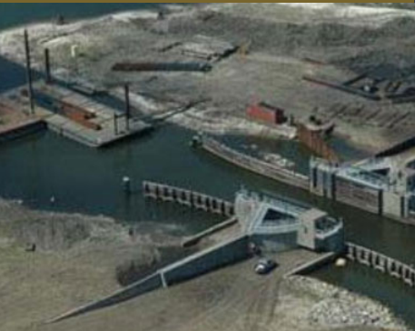
Bayou Dupre Sector Gate Control, Structure Reach LPV 144, New Orleans, Louisiana Flood Control and Hurricane Protection Infrastructure post-Katrina.
